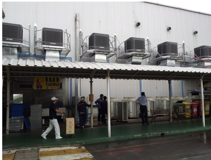
Example of evaporative fan (MUK) those are installed in a factory
